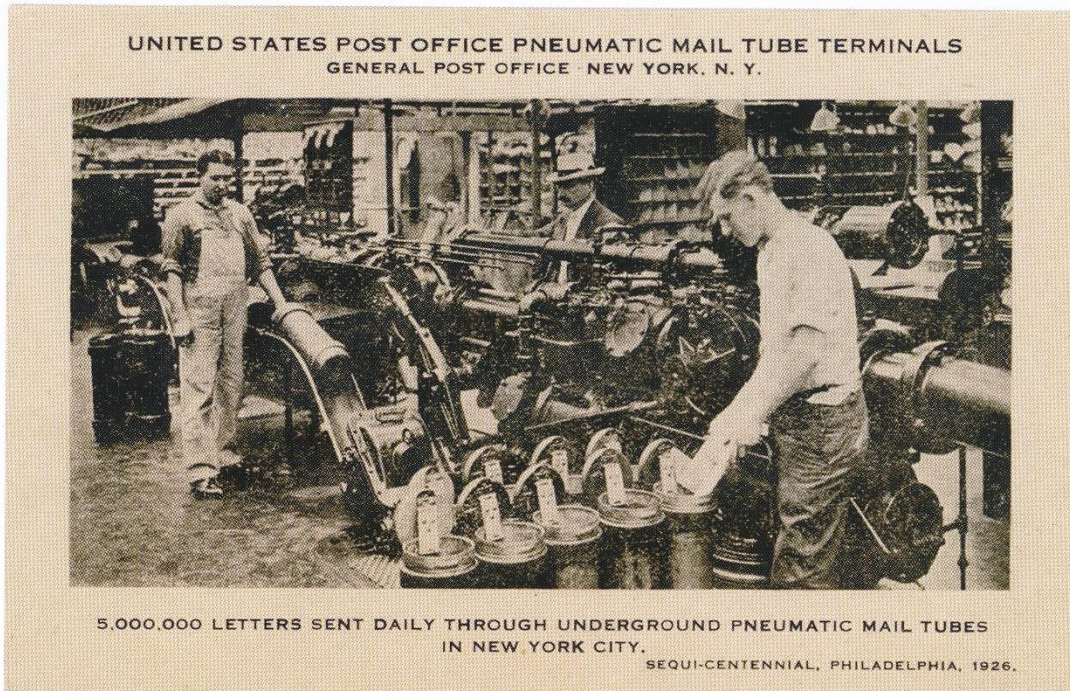
Figure 8. Operators at pneumatic sending and receiving apparatus.
